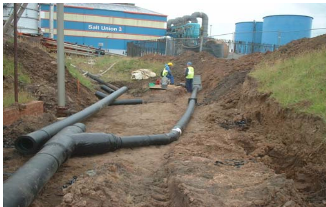
Main pipe splits into 10" & 8" to connect into steel main.
